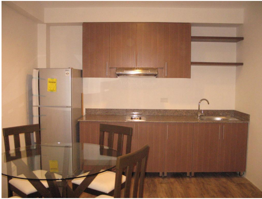
Granite kitchen counter fitted with laminated overhead & base cabinets
