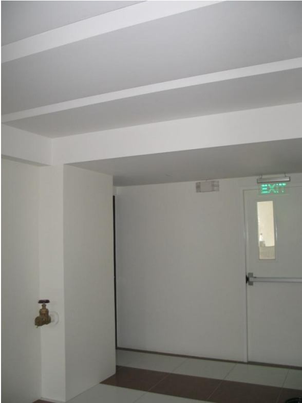
Fire exit @ the hallway
